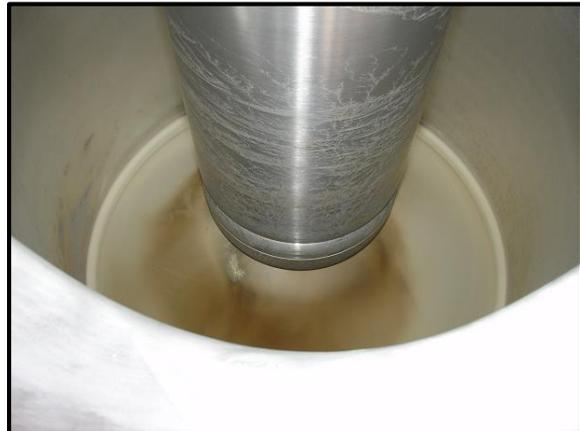
Below is shown a case where the breaker required many fills over its 35-year life. The leak site admitted enough water over the years to cause the center phase to flash-over; and internal phase to ground fault.
